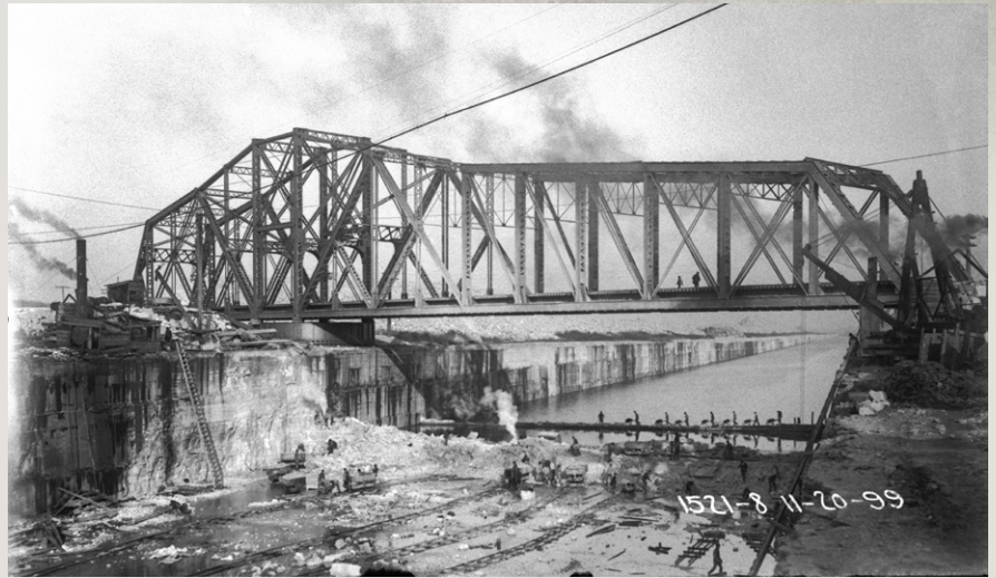
A line of workers move rubble during construction of Chicago Sanitary & Ship Canal, 1899, at Lemont Railroad Bridge. The canal cut through Silurian-age limestone bedrock.
