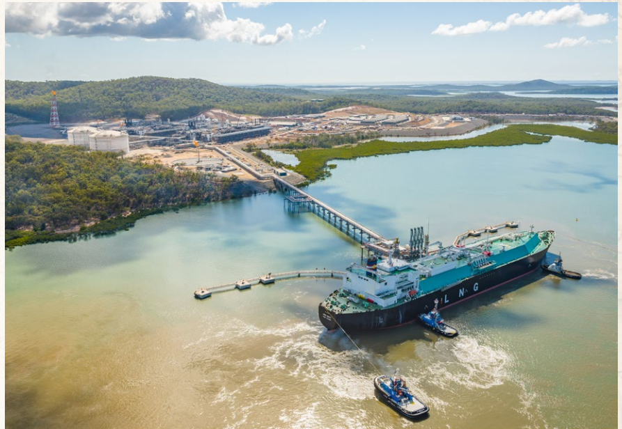
Curtis Island Liquefied Natural Gas facility in Queensland, Australia.
